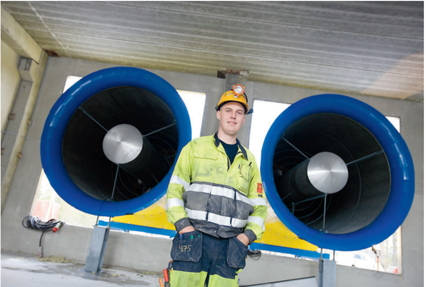
A lot of air is needed down in the mine. Large fans press down fresh air a thousand meters using ABB's Automation System 800xA. "It works very well," says Emil Fjellner, electrician at the mine in Kristineberg and person responsible for the ventilation system.
