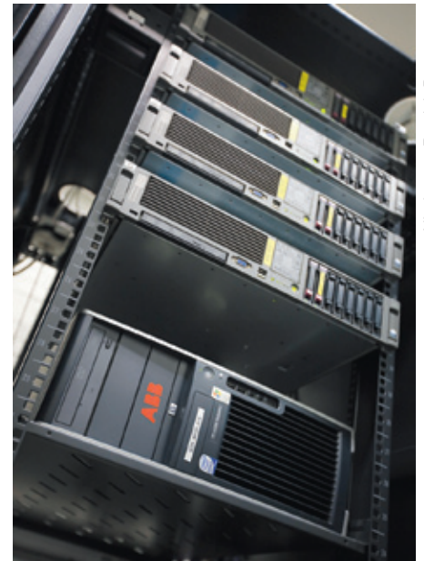
System 800xA is discrete but an effective “brain” in the Kristineberg mine ventilation system.
