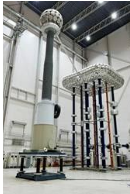
Fig 3. Testing of transformer bushing
