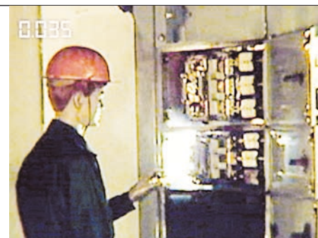
1b Arc accident with ABB's ArcGuard System™
