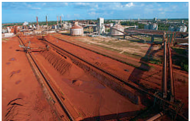
4 Alunorte plant in Brazil.
