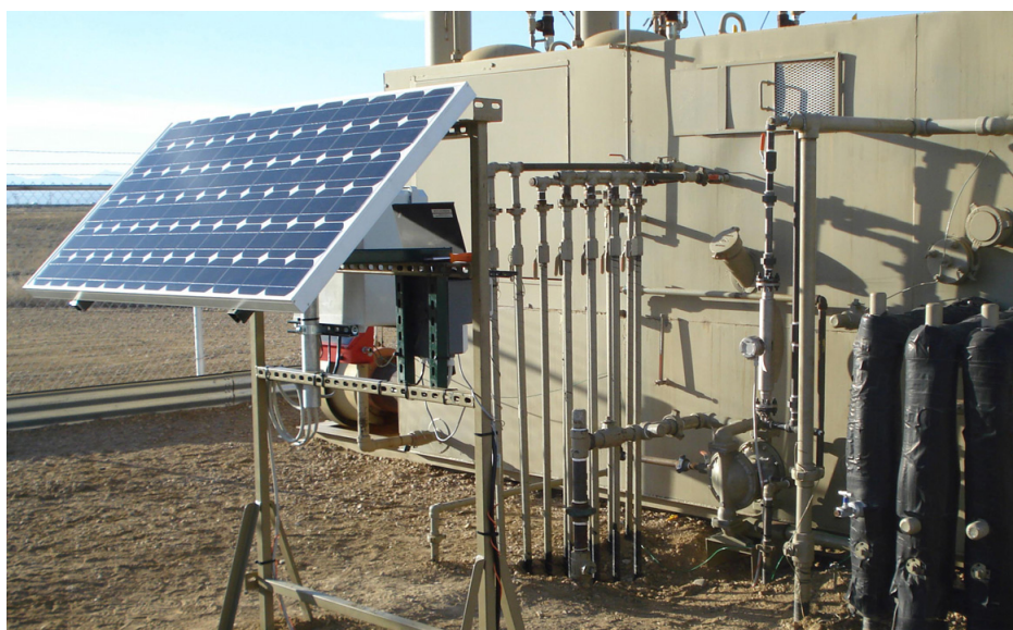
Fig. 6: Totalflow XRC 6490 G4, Modbus RTU communication and solar panel for power supply
