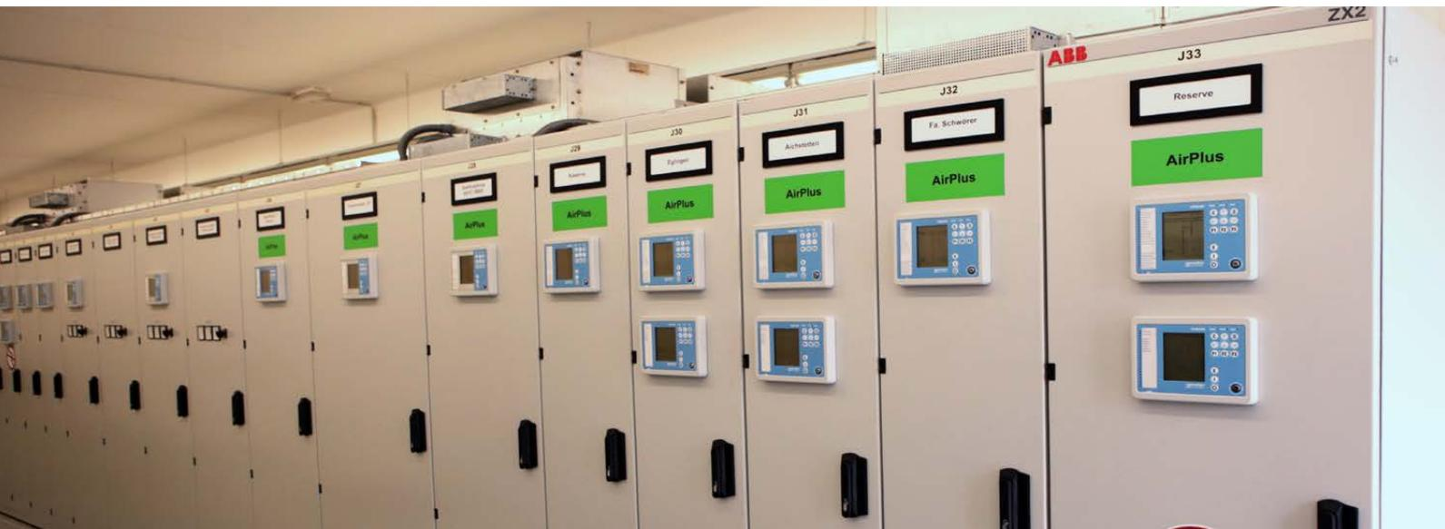
01 The dimensions of the ZX2 AirPlus panels are identical to conventional ZX2 panels and follow the same operation scheme. An ideal setup for the customer to compare both technologies side-by-side in real life operation.
