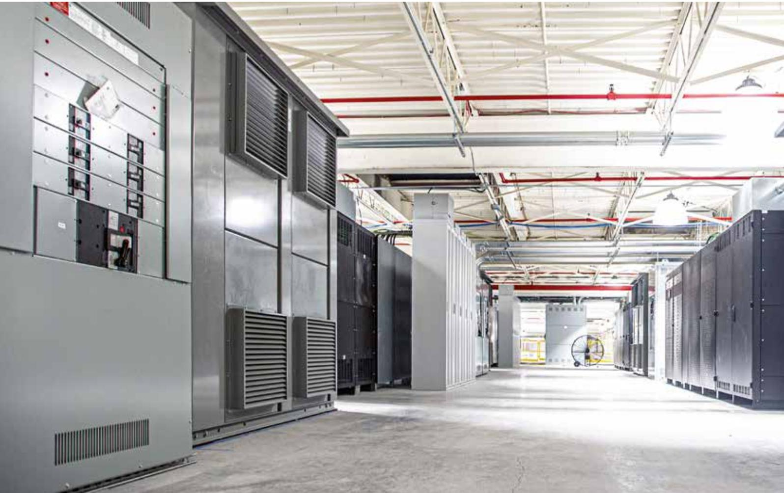
— 01 ABB and GIGA Data Centers developed an electrification solution of LV switchgear, dry-type transformers and UPS to support the IT server and network infrastructure of the GIGA Data Centers is shown.
