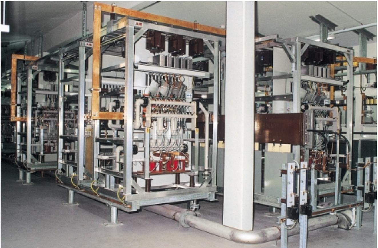
controlling chokes; hence, the 'external' circuit-specific losses (which are recoverable at the cost of additional circuitry) are not considered in the thermal budget of the device. In the conducting state the IGCT is a *thyristor* with two injecting emitters giving it half the conduction loss of a transistor structure and allowing more room in the thermal budget for dynamic losses, and hence for frequency.
