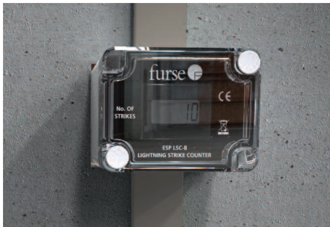
Furse ESP LSC-B secured to down conductor of building's lightning protection system
