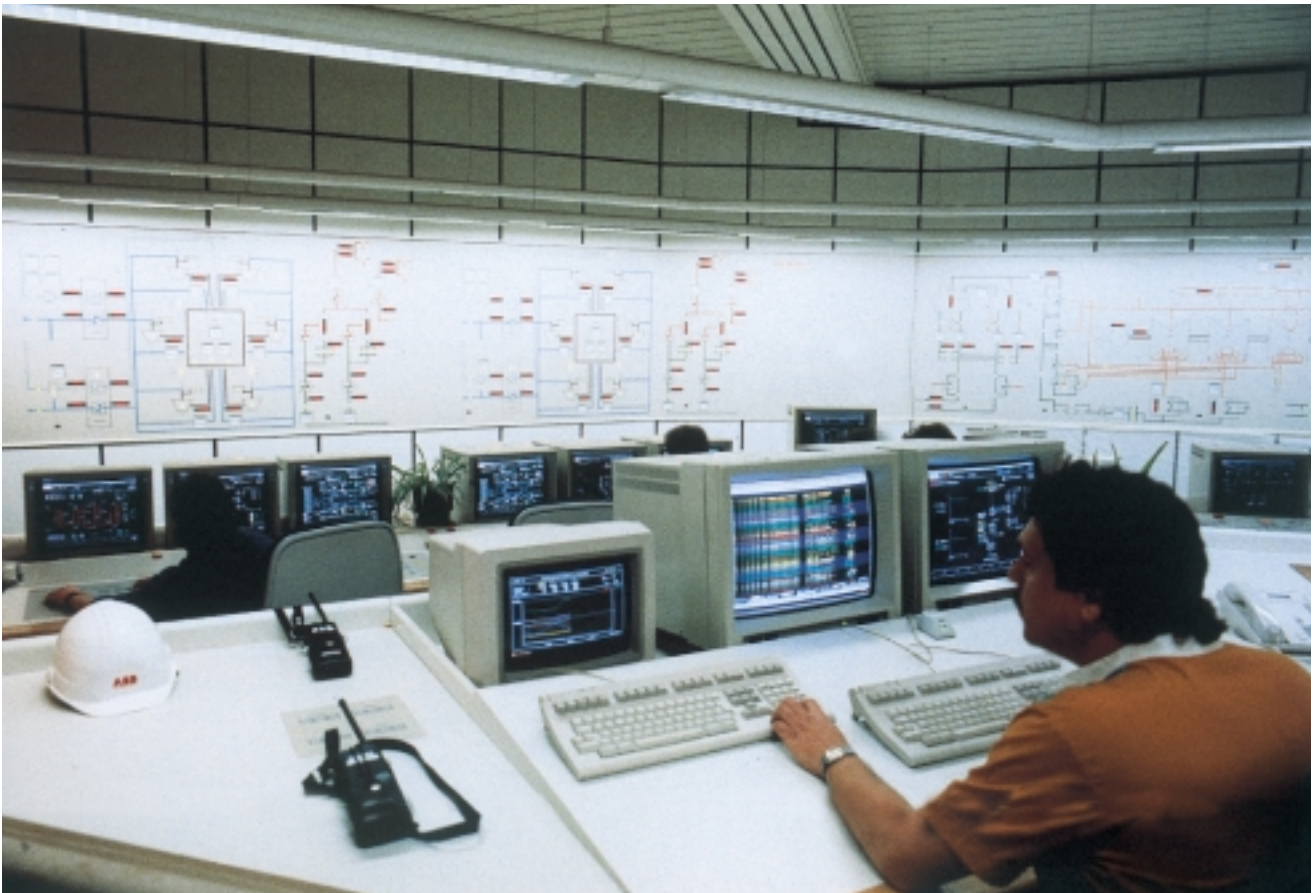
Dual-unit control room after the total renewal of the control system. Conventional back-up instrumentation was reduced to an absolute minimum. All the original distributed control rooms are now concentrated in the new control room. 8
