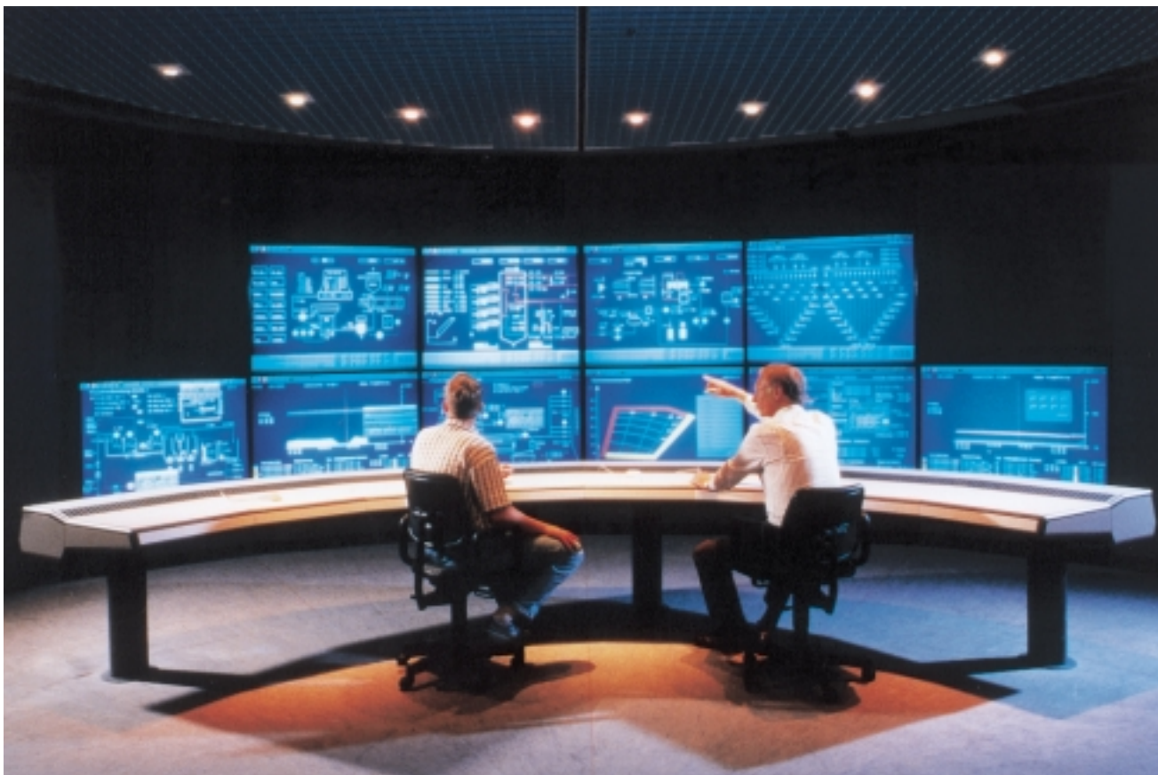
Advanced twin-unit control room in the 900-MW Schkopau power plant
