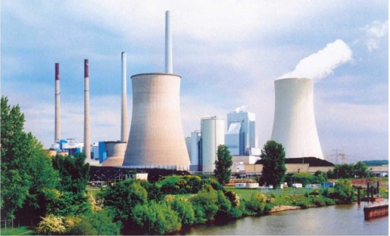
A refurbishment project – the 2 × 250-MW Staudinger coal-fired power plant in Germany
