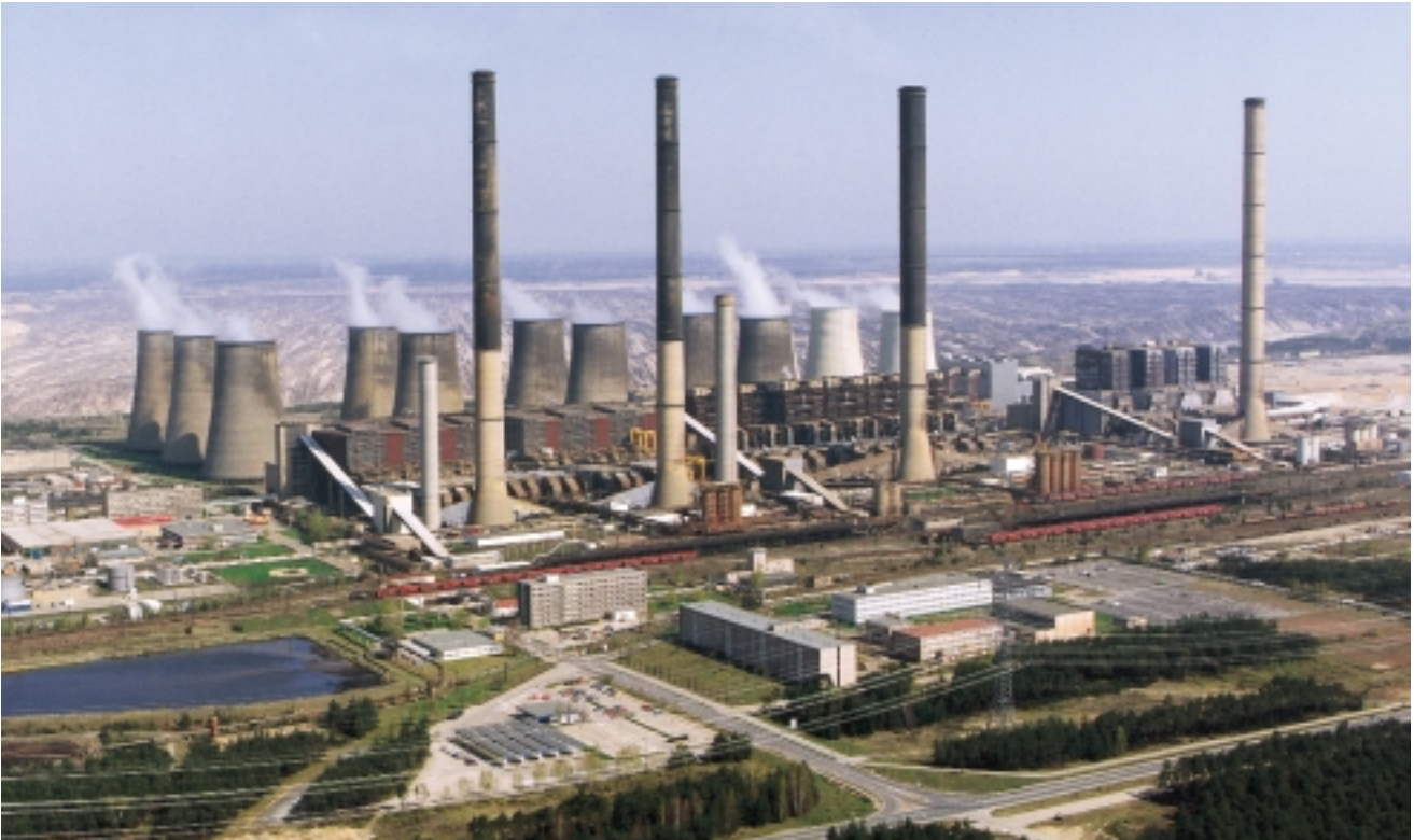
Refurbishment project at Boxberg, Germany, where a 2 × 500-MW lignite-fired power plant was upgraded
