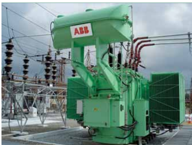
3 The newly revamped BIOTEMP® vegetable oil filled transformer in operation at a CEMIG substation bay
