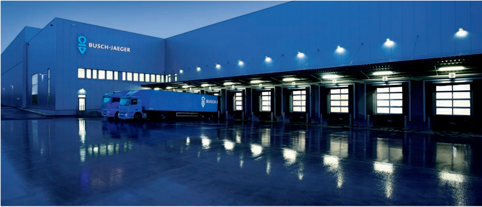
Logistics Centre at the headquarters in Lüdenscheid
