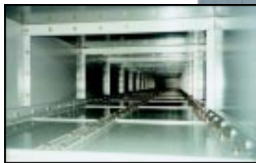
Plenum provides escape route for gases and protects people, equipment and PDC.
