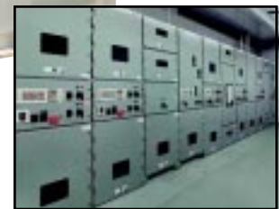
Primary and secondary equipment including control systems install in a PDC for turnkey delivery of a unit substation.
