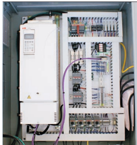
2 ACS800-U11 line-regenerative drive. Photo © Uni-Systems
