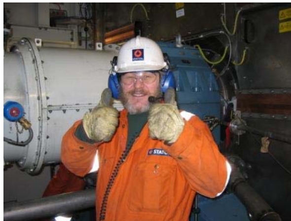
Statoil employee at Troll A signals successful conclusion of commissioning tests. HVDC Light's offshore converter, named Electronic Drive System or EDS module, directly drive newly installed nearly 55'000 HP gas pre-compressors.
