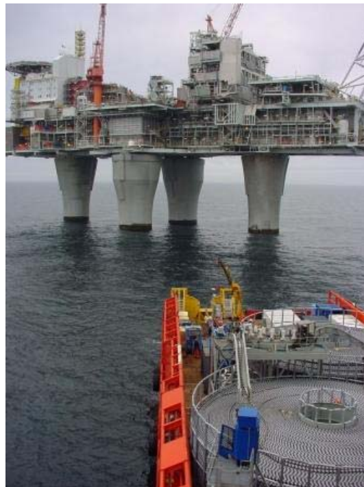
Loaded on a cable-laying vessel, ABB's subsea cables arrive at Troll-A having carried out installation operation on the seabed by conventional submarine operation along the 70 kilometer distance. The cables are protected by water jetting into seabed or by rock dumping.
