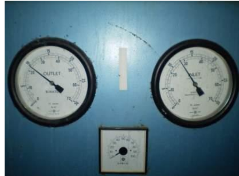
Sand Filter Pressure
