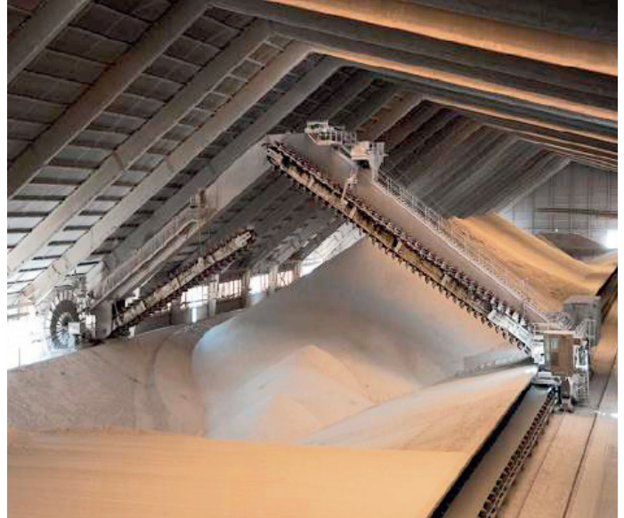
Raw material stockyard with reclaimers
