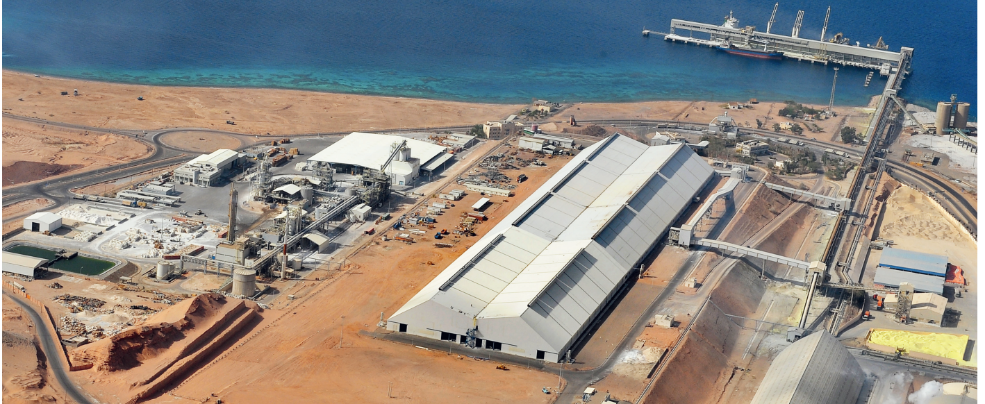
Arab Potash Co. (APC) plant in Jordan
