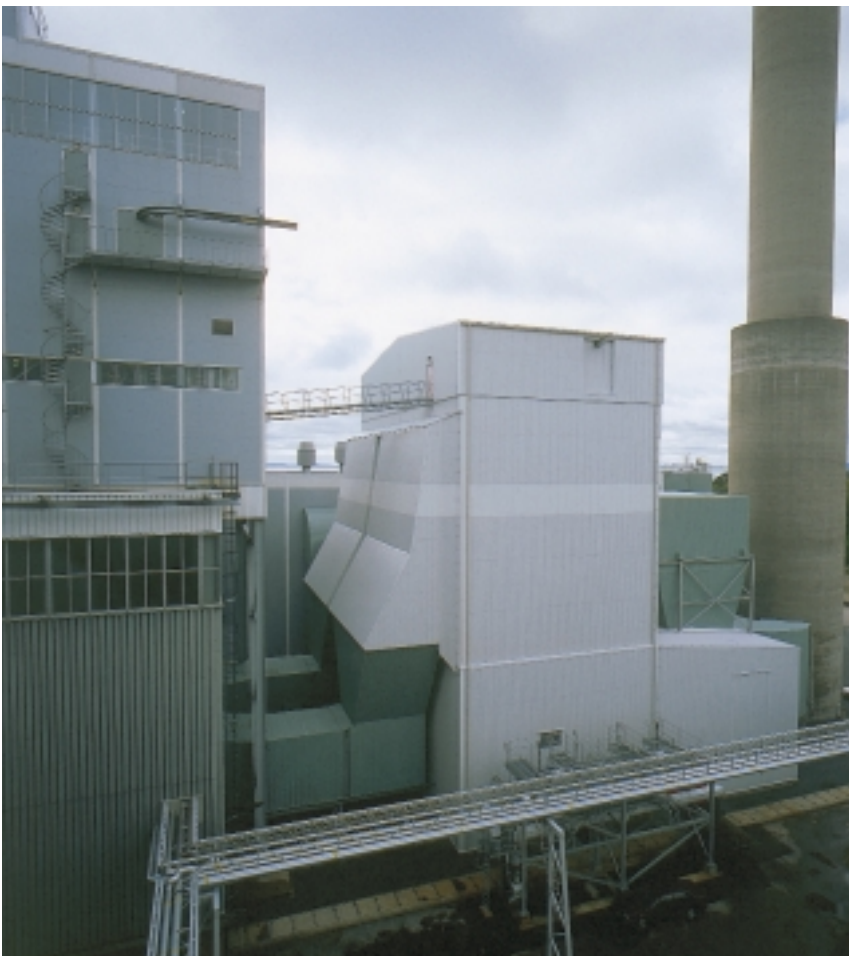
New electrostatic precipitator from ABB in the 20-years old Karlshamn oil-fired power plant, Sweden. The precipitator began operating in 1997.
