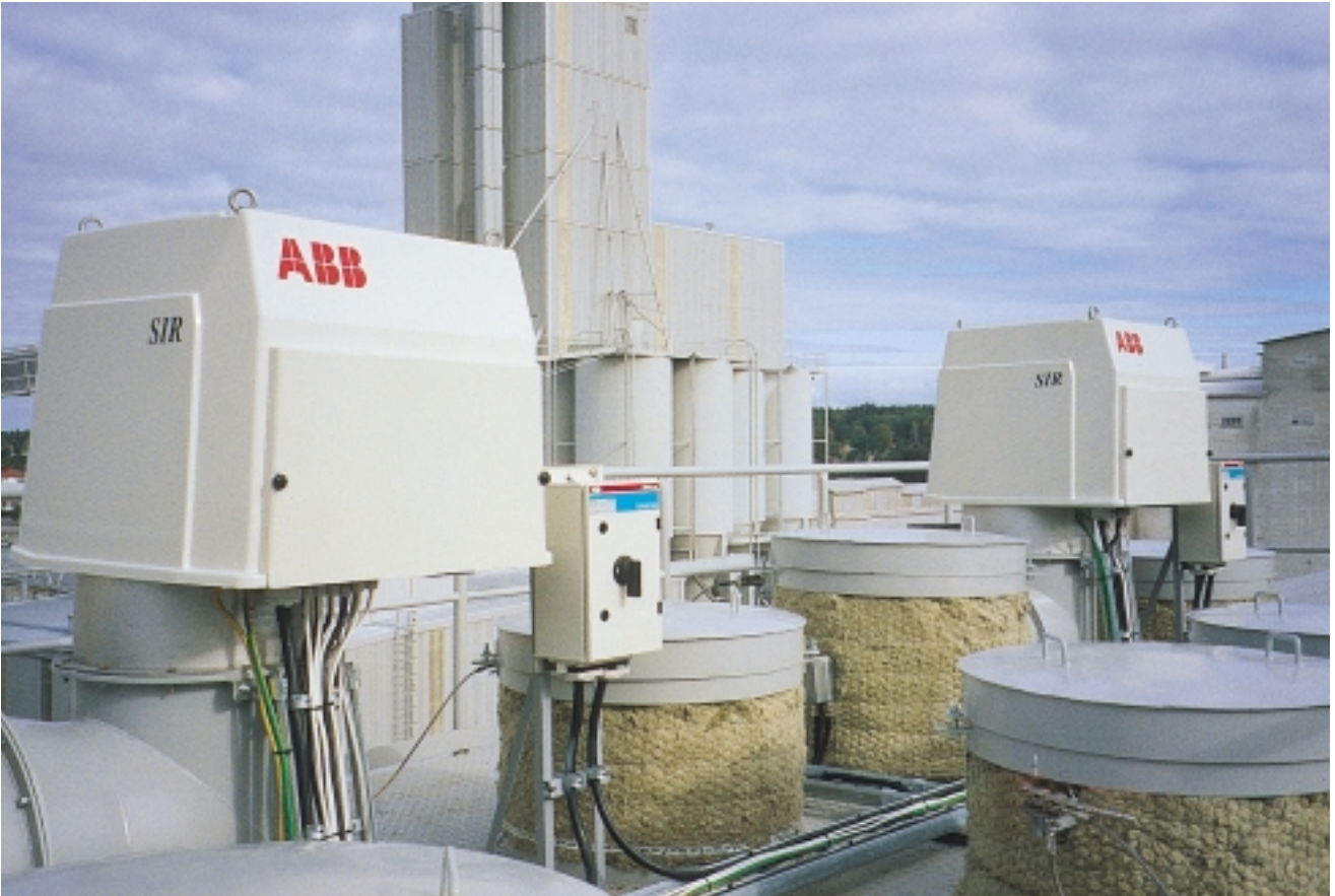
Two SIR units on the roof of an electrostatic precipitator. Due to their low weight, the units can be mounted directly on the tubular encapsulation around the high-voltage feeder.
