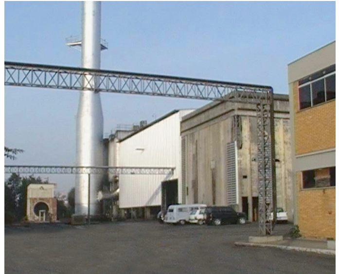
SSB Energia Renovável's plant in Limeira uses wood chips to produce steam for industrial processes.
