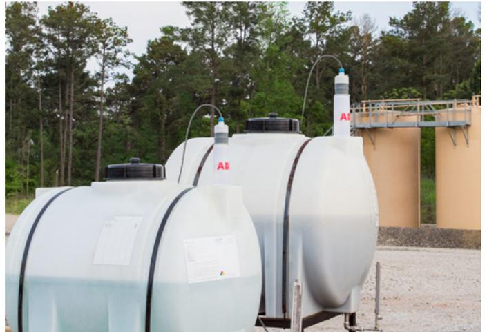
Fig. 2: LST100 mounted using the mounting bracket
