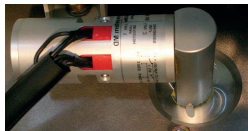
Fig. 7.12.3: Signal lamp for gas density (used when the signal is not integrated in the protection device)
