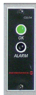
Fig. 7.12.3: Signal lamp for gas density (used when the signal is not integrated in the protection device)
