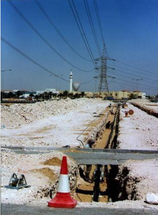
Fig. 5: Example of cable laying in a corridor already used by OH-lines. AC PEX-cable in Qatar.
