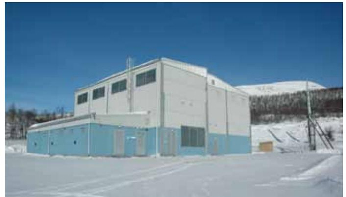
Figure 8. Example of 145 kV indoor substation with DCBs.
