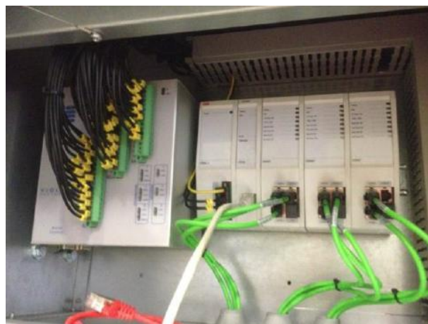
Figure 5. RIO600 as fault passage indicator with remote control.
