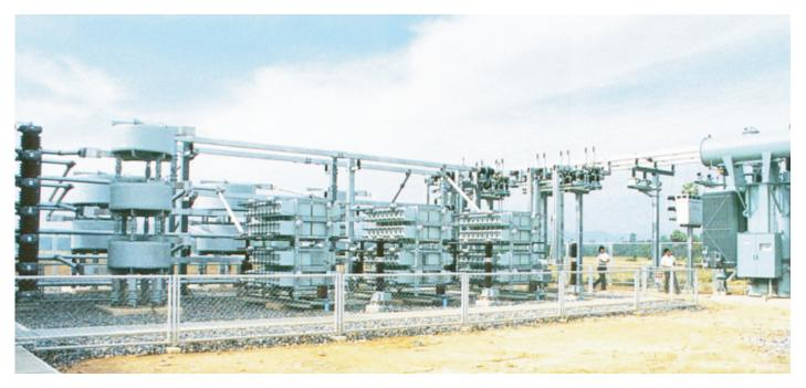
To improve the voltage control and stability on the Central Southern 115 kV tie line the Electricity Generating Authority of Thailand (EGAT) is operating a Static Var Compensator (SVC) at Chumphon Substation. This SVC was supplied by ABB and has been in operation since 1987. The dynamic operating range is from 60 Mvar capacitive to 20 Mvar inductive.
