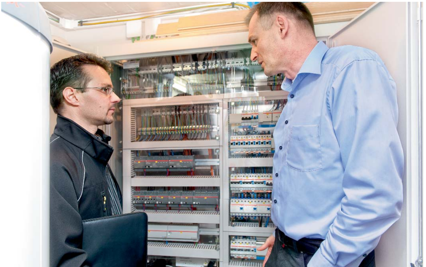
Electrician Roger Acklin (left) and homeowner Dieter Kunert installed functions, such as the light and temperature regulation systems, via a central switch cabinet in the cellar.
