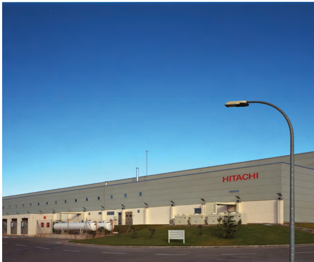
Hitachi Air Conditioning Products Europe - HAPE Production facility - Barcelona, Spain
