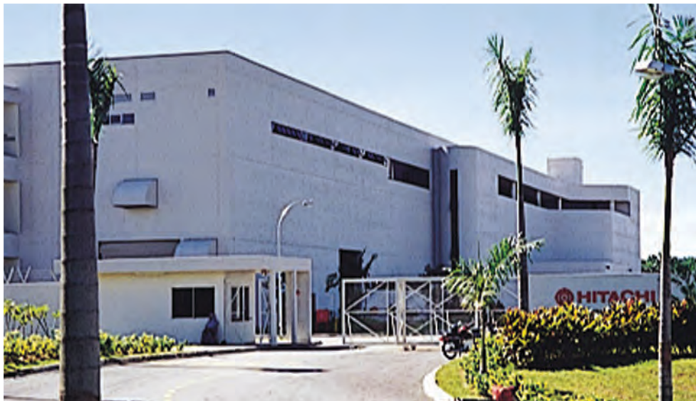
Hitachi Air Conditioning Products (M) - HAPM Production Facility - Kuala Lumpur, Malaysia
