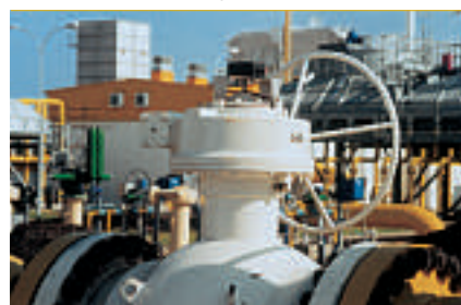
5 Hand operated cut-off valve for one filtration pipe string.
