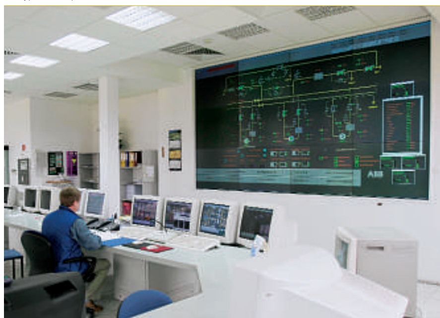
4 Typical compressor station control room.
