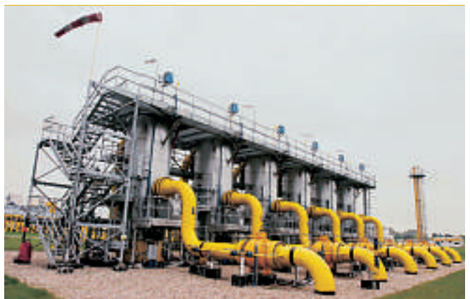
3 Gas filter station.
