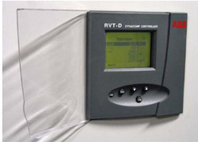
Figure 45: RVT-D controller installed in door panel RVT-D 门板安装前试图
