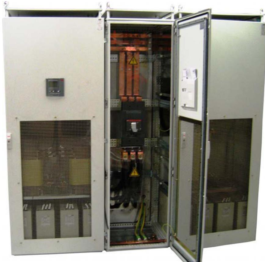
When a single connection point is requested, the cable entry cubicle can be located in several places, as shown in [Figure 18](#) with a two cubicles DYNACOMP. 当选择单独连接点，电缆进线柜可以放置到几个地方。如图 18 所示带有 2 个单元的 DYNACOMP.
