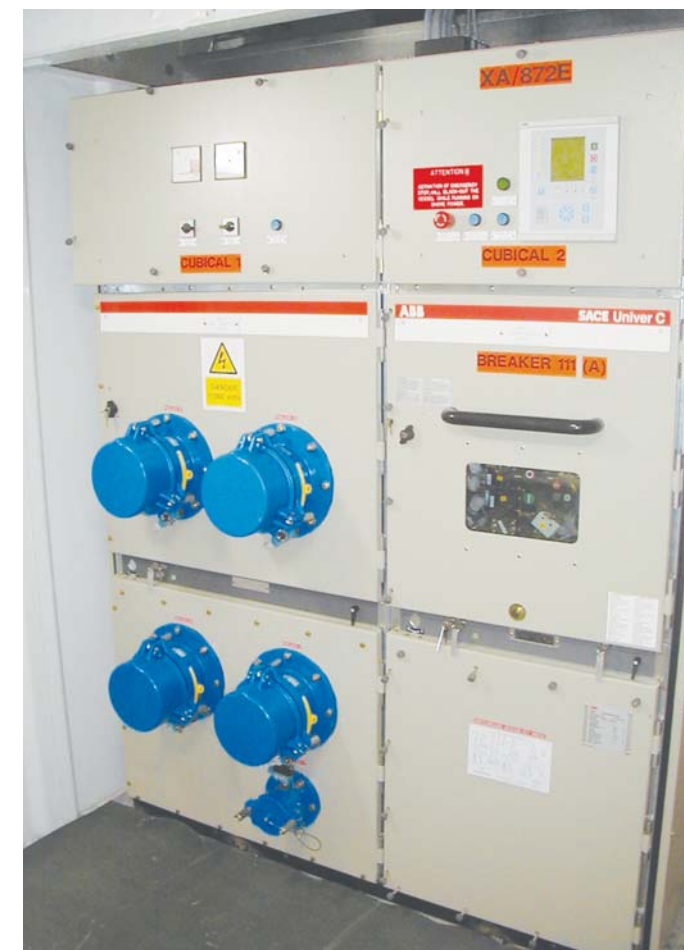
Figure 2 shows a ship with diesel machinery and low voltage electric system. The shore-to-ship power system is arranged with the shore connection panel located outside the main switchboard room with cable connectors mounted in the front. An onboard transformer steps down the power from high to low voltage.
