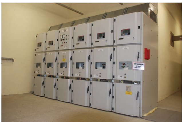
Medium voltage distribution system.
