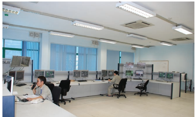
Central control room at Cam Pha.
