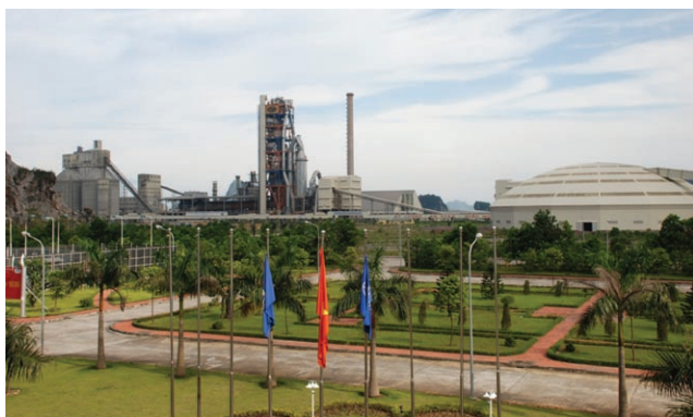
Cam Pha Cement plant.
