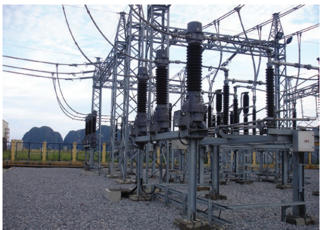
High voltage distribution system.
