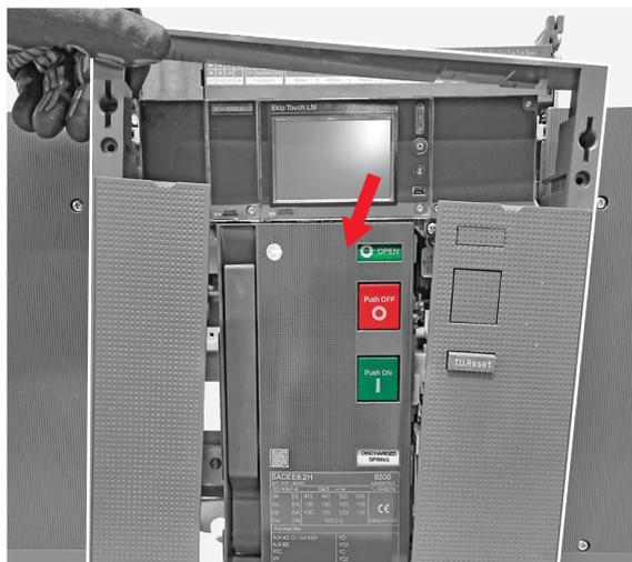
**6** By means of the torx key unscrew the 2 screws fixing the 2 plugs to the front cover.
