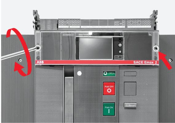
**2** Manually remove the trip unit transparent cover.
