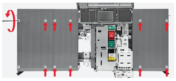
**18** Manually remove the left shields.
