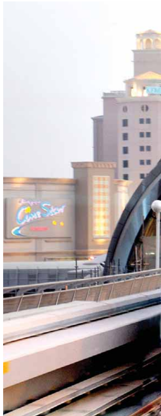
ABB powers the Dubai Metro
