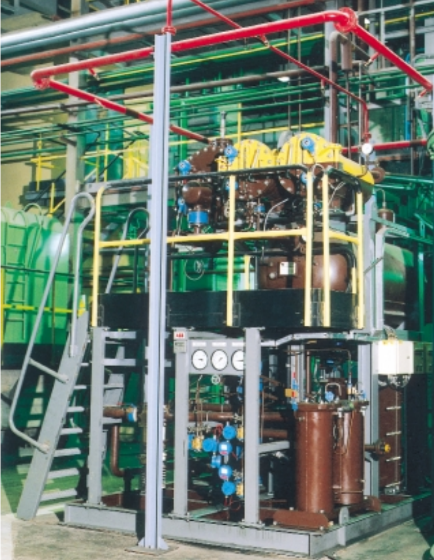
New seal oil unit installed at Dolna Oldra power plant in Poland. The system comprises a single unit, and all accessories are located in one place. Connections to the generator are direct.
