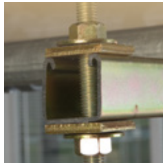
Standard method using nuts and washers.
