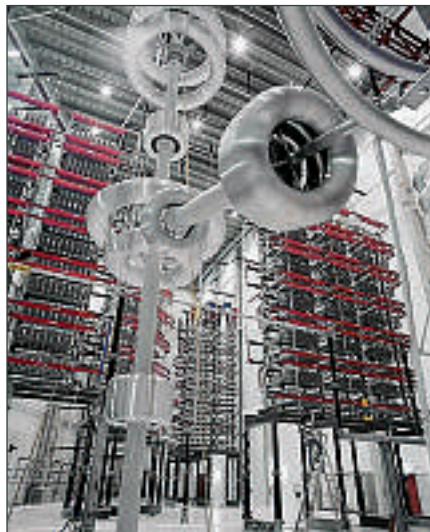
1 Capacitor banks in the voltage section of the synthetic circuit
