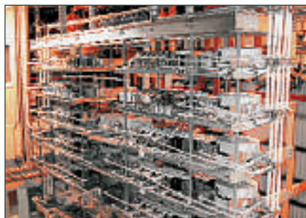
2 Six-pulse back-to-back bridges and test object used in the new synthetic test circuit
