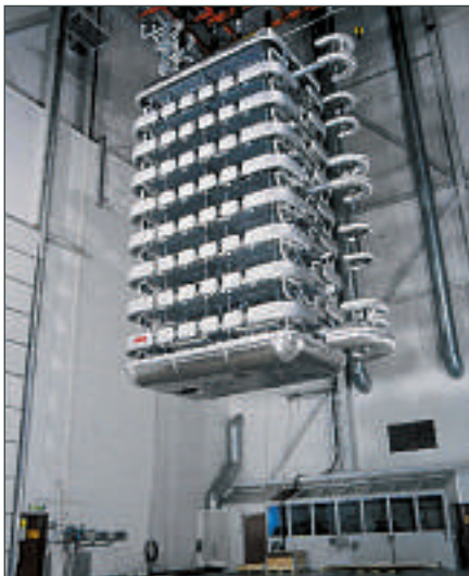
6 A double valve structure for the Three Gorges – Changzhou HVDC project in China.
