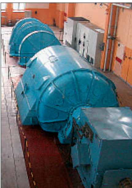
3 The test circuit generator, supplying continuous test currents of up to 4000 A_{rms} at 50 Hz
