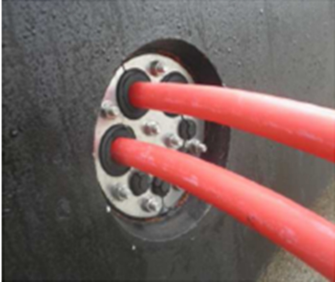
Fig. 9 : sealed cable entry
