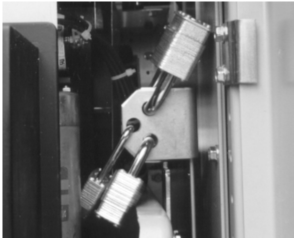
Fig. 7-6. Test & disconnect position padlock device (WP-08/16/20 and WPF-08/16 breakers)
