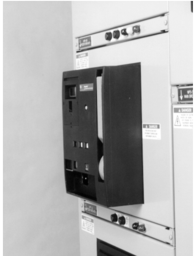
Fig. 5-9. Push the breaker in completely. Close the door.
