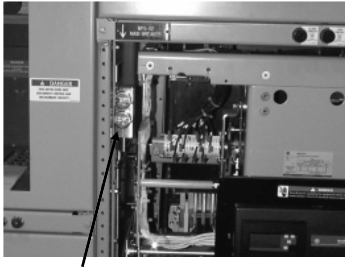
Fig. 5-21. Key is captured in key interlock until breaker is opened
