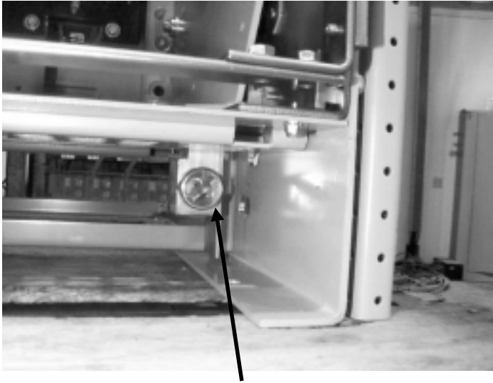
Fig. 5-20. View showing FRE key interlock locking FRE in connect position
