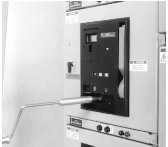
Fig. 5-10. Engage the racking screw with the racking handle (WP-08/16/20)
