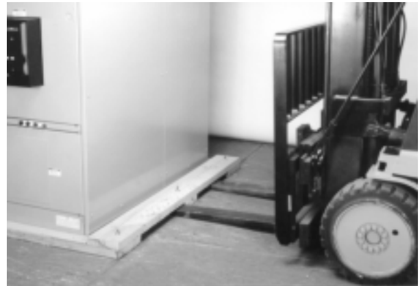
Fig. 2-6. Placing forklift tines under AKD-10 equipment shipping skid
