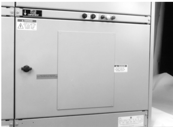
Fig. 7-4. Future-use breaker compartments
