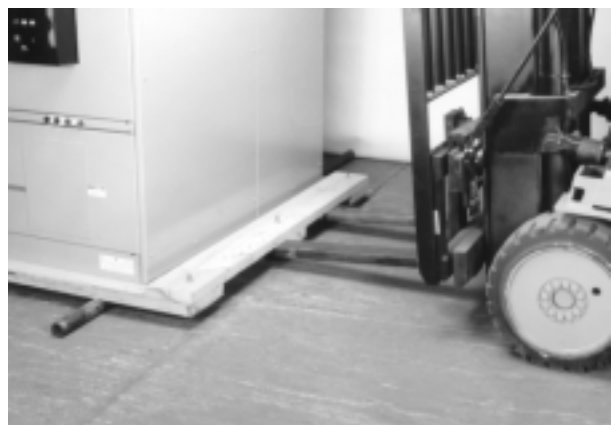
Fig. 2-7. Placement of rollers under shipping skid
