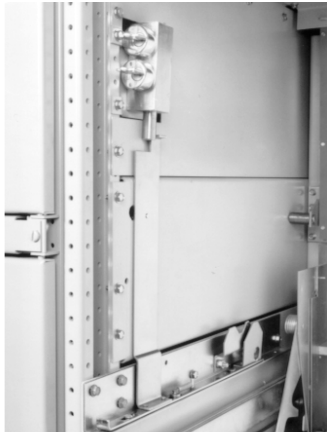
Fig. 7-5. View showing circuit breaker key interlock to provide protection against unauthorized operation
