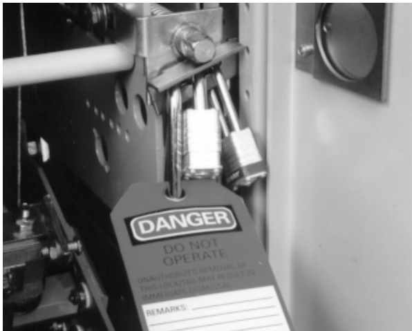
Fig. 7-7. Racking mechanism padlock device (WPS-32/40/50 breakers)
