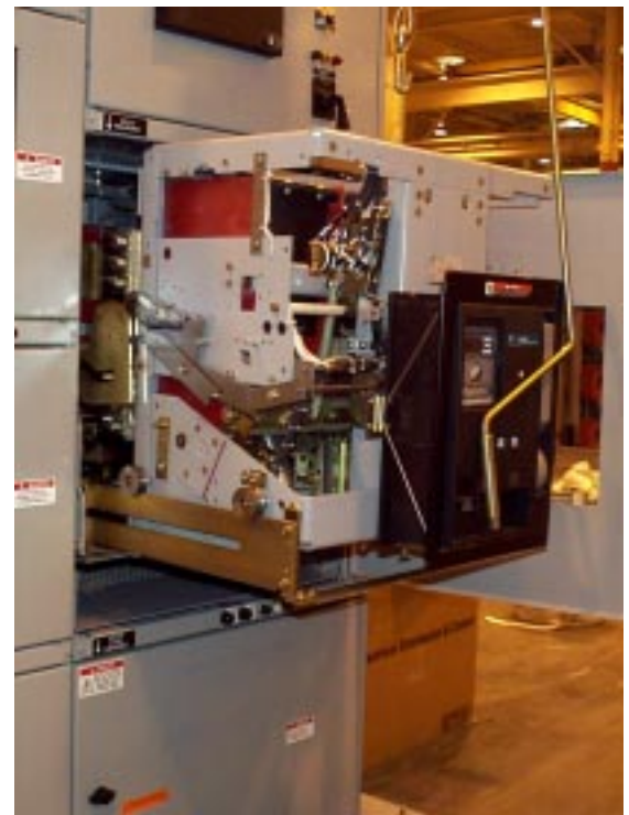
Fig. 5-8. Lower the breaker onto the rails of the cell. Remove the spreader bar assembly
