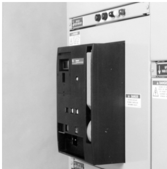
Fig. 7-1. WavePro switchgear circuit breaker shown in DISCONNECT position
