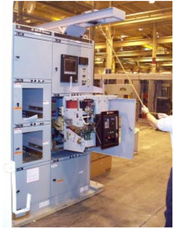
Fig. 5-6. Hoist breaker above rails
