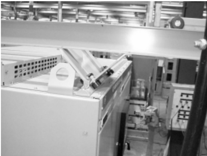
Fig. 4-27. Front rollers positioned on front track
