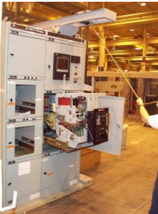
Fig. 5-7. Pull rails out completely from the circuit breaker compartment
