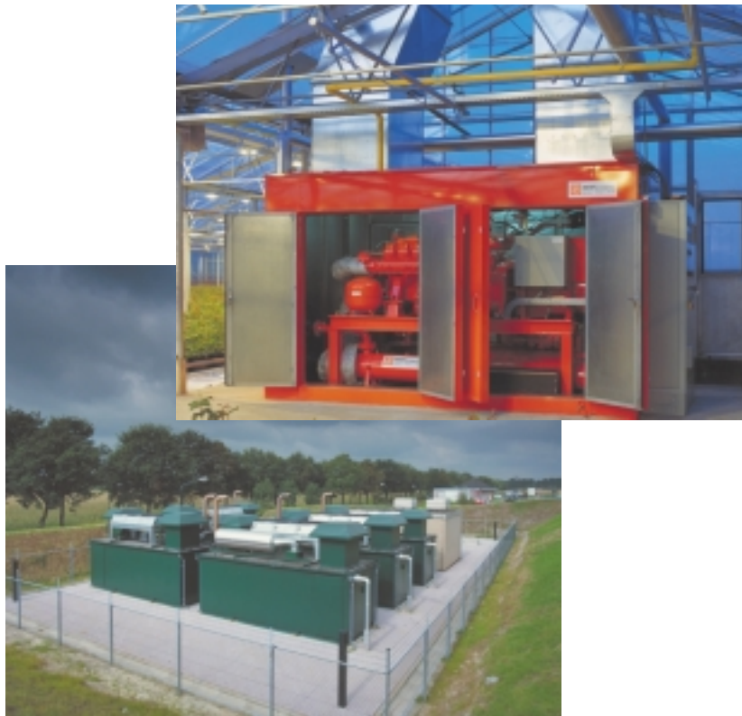
Cogeneration of heat and power improves the overall energy efficiency even further.
