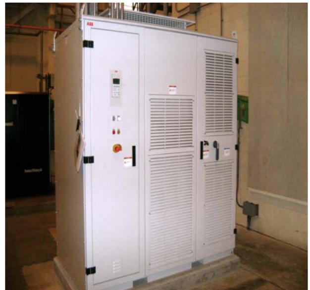
**ABB ACS 2000, 4160 Volt, Direct to Line, 600 hp VFD at Beloit**
