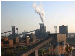
Integrated Steel Mill, Southern Europe
