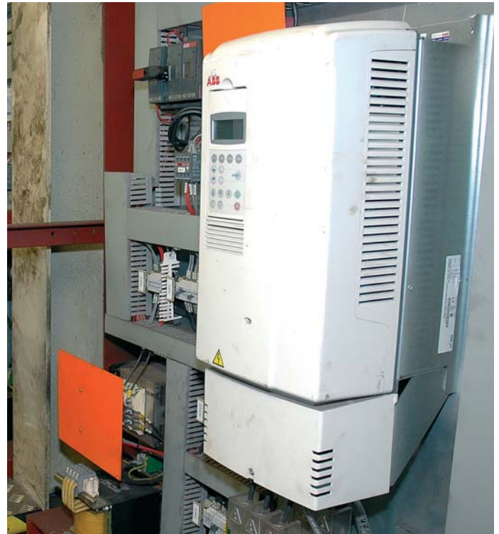
One of several 200 kW ABB industrial drives used by Carinox.
