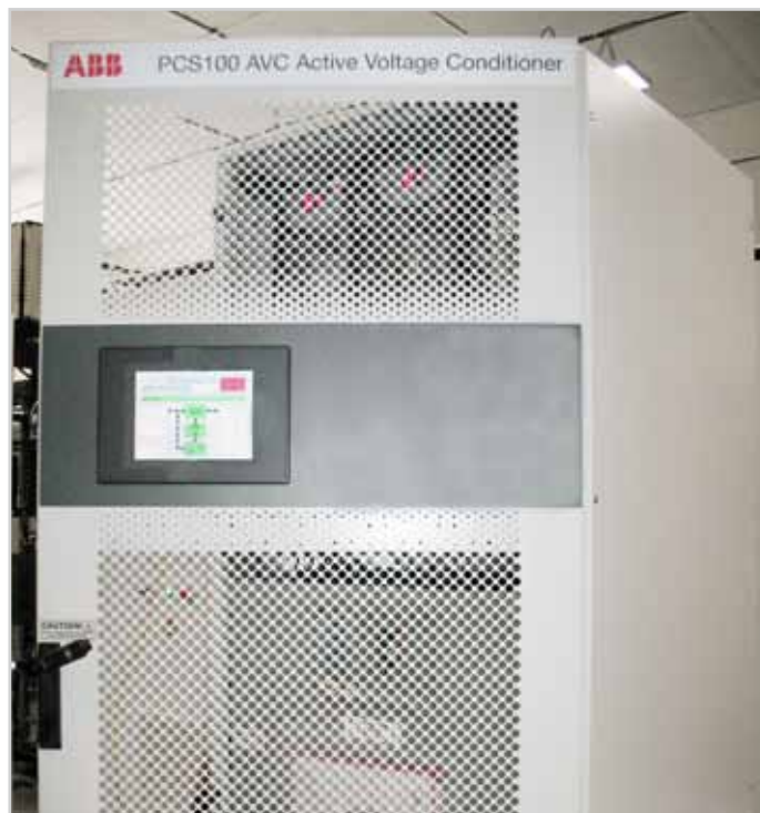
ABB's PCS100 Active Voltage Conditioner installed at Gubkinskiy GPP
