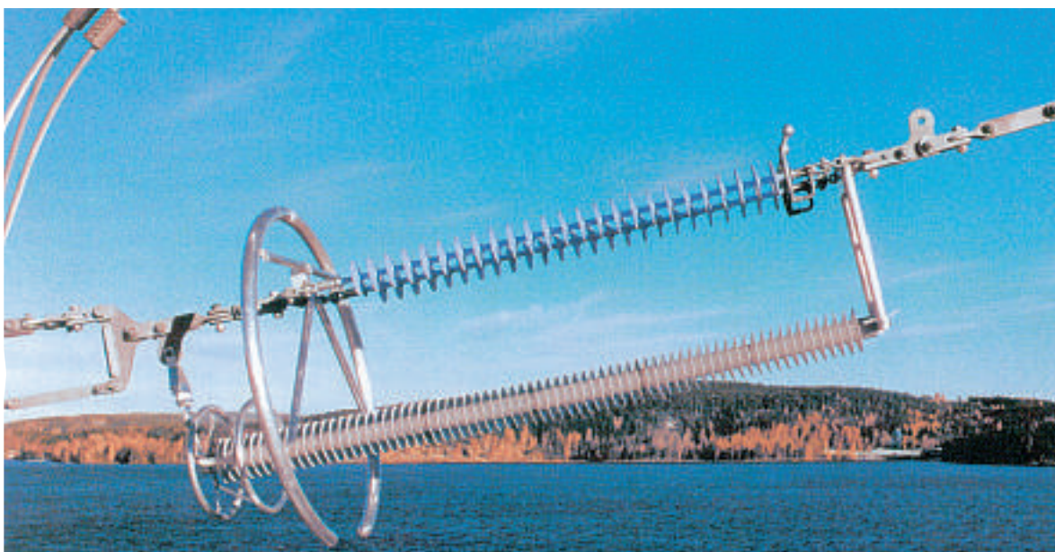
1 Line surge arrester across a 400-kV tension insulator string. A disconnector is at the high-voltage end, to the left.
