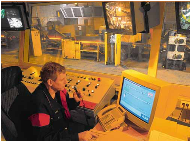
1 Operator's booth with control and monitoring equipment
