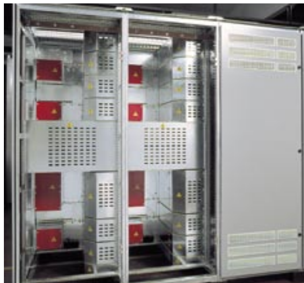
Representation of the structural frames in form 3a, 3b and 4b for switchgear type PC3.0/MNS R
