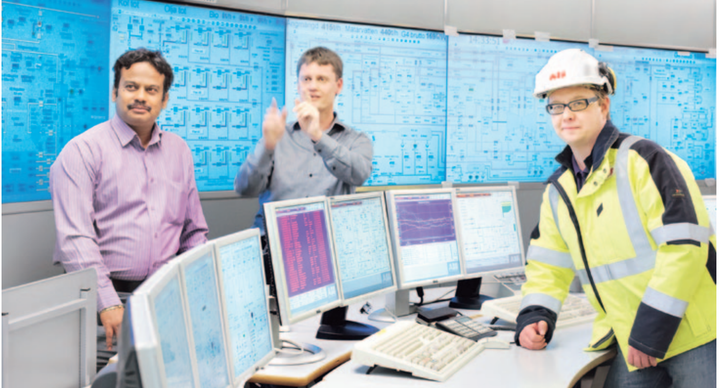
Virtualization replaced thirteen physical servers with two. Three of the virtualization project team members gathered in the plant's main control room. From the left: Krishna Kumar, ABB, Kjell Thuné, Mälarenergi, and Jonas Gustavsson, ABB.
