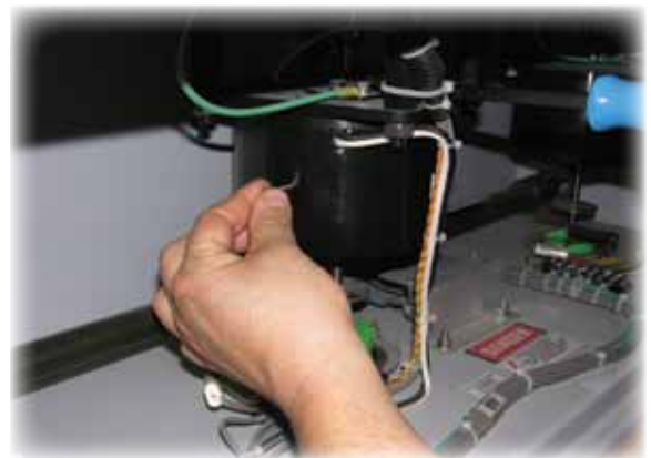
Wear indicators provide simple go / no go indication when interrupters need replacement, eliminating maintenance.
