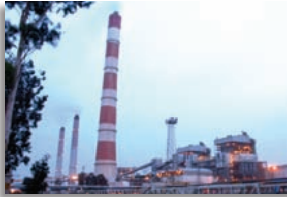
NTPC Vindhyachal stage I, 6 X 210 MW
